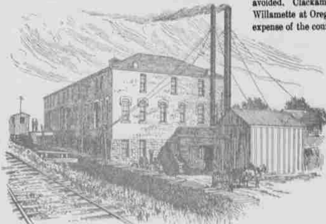
AGRICULTURAL WORKS AND ELECTRIC LIGHT PLANT, SALEM.
