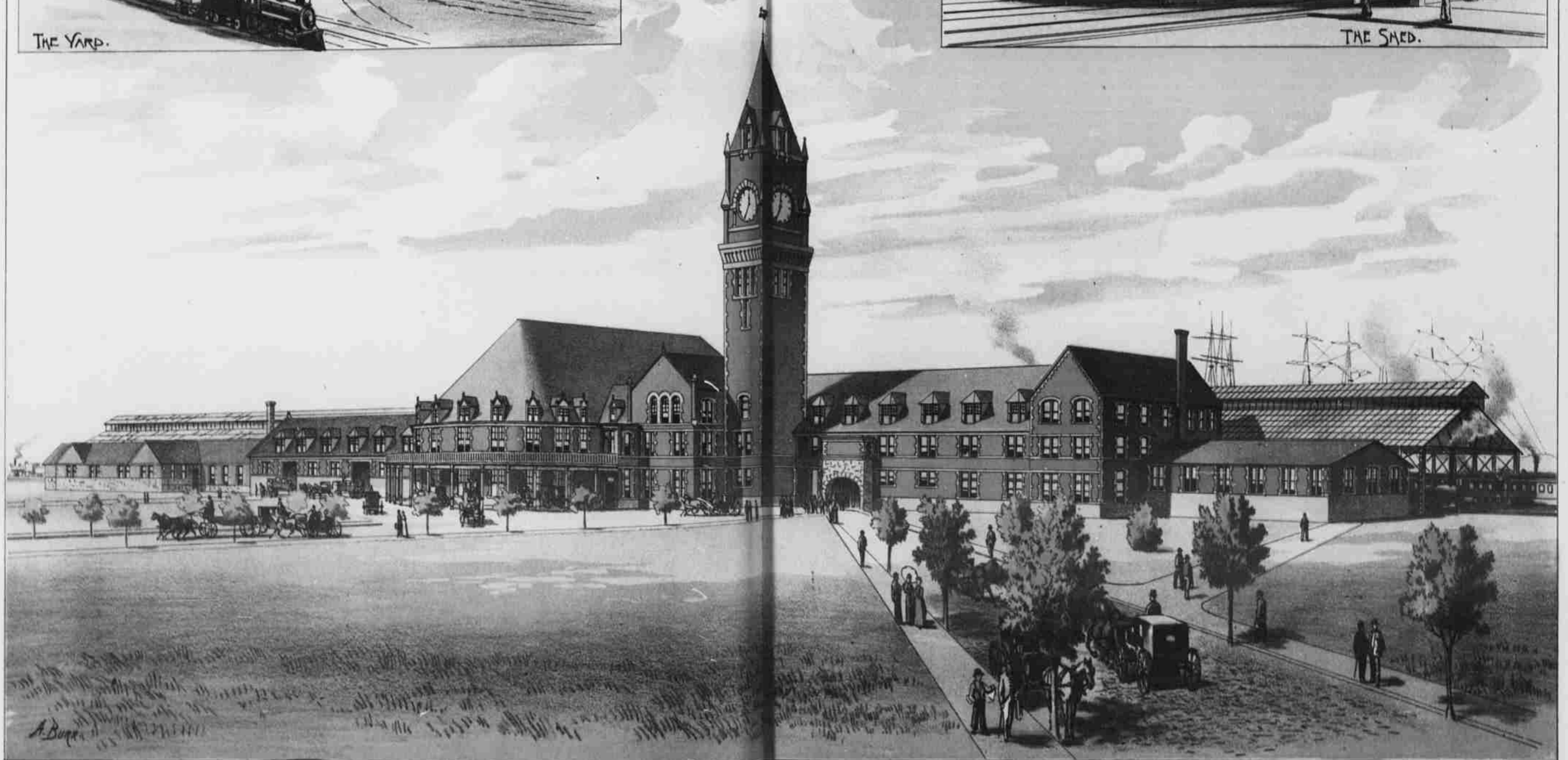
OREGON—THE MILLION DOLLAR UNION DEPOT UNDER CONSTRUCTION AT PORTLAND.—See Page 3.
