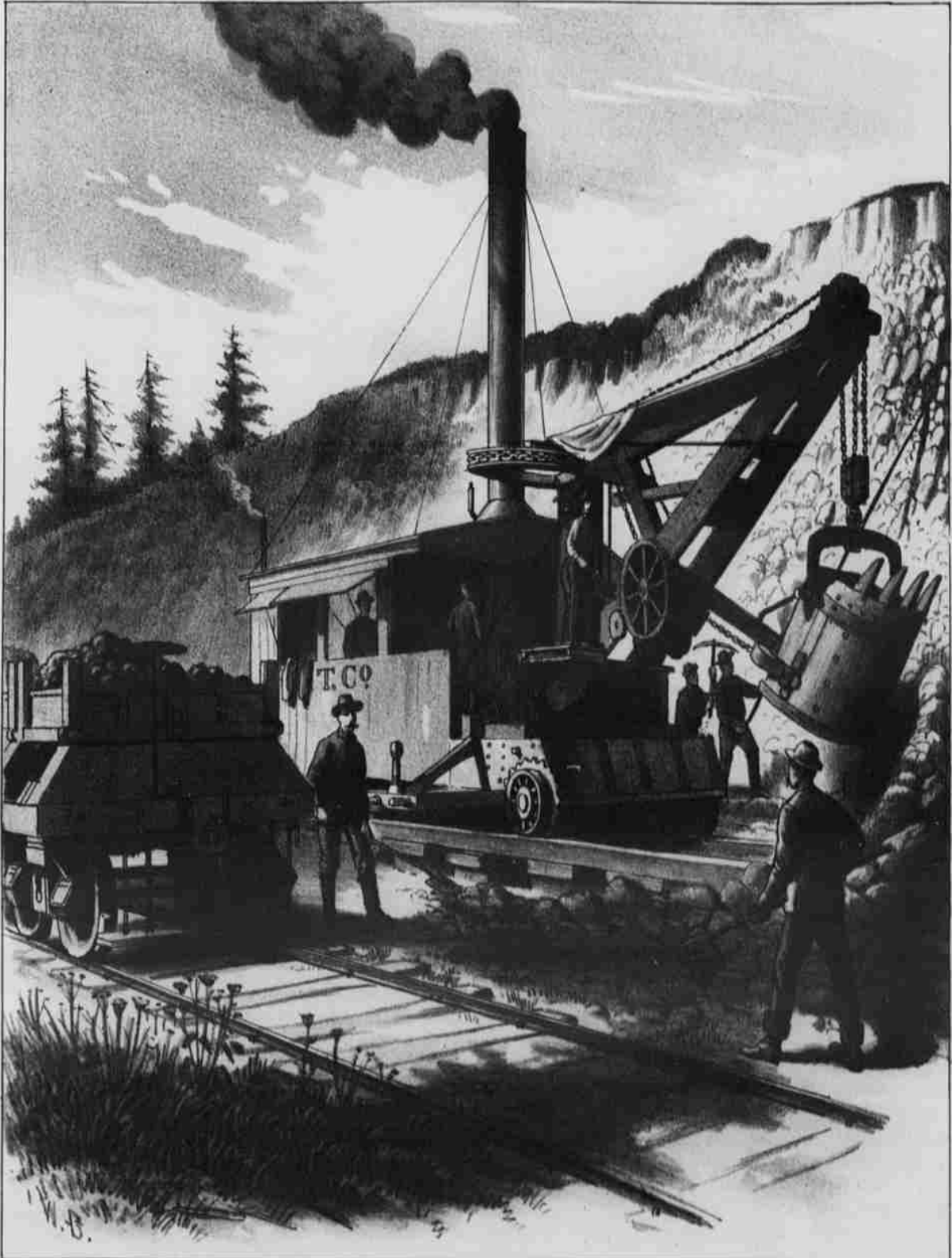
OREGON—Steam Excavator at Work for Portland's Union Depot.—See Page 3.
