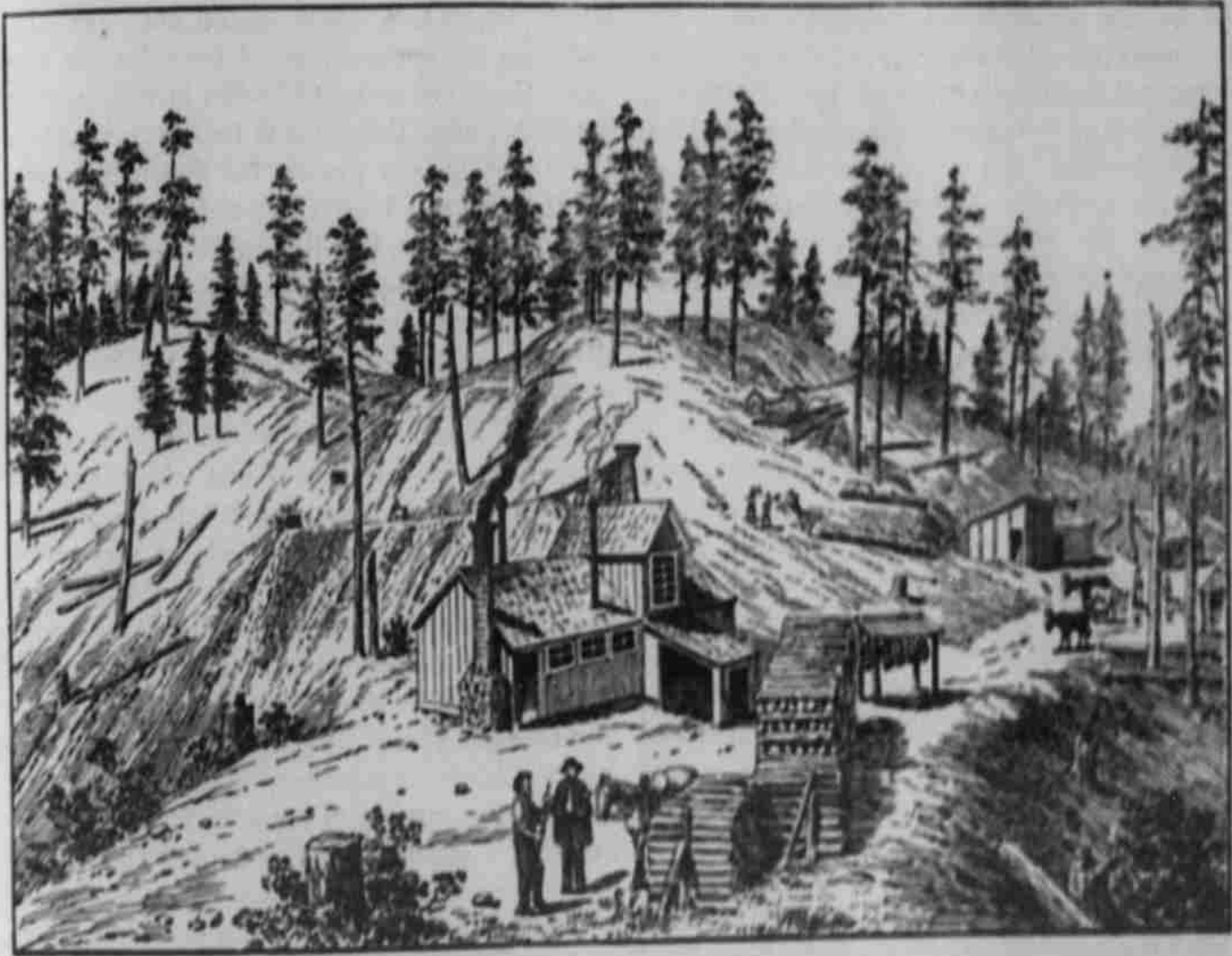
ELK HORN, FIRST QUARTZ MILL ERRECTED IN IDAHO, NEAR IDAHO CITY.
