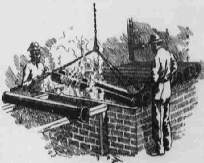
DIPPING PIPE IN COAL TAR.
