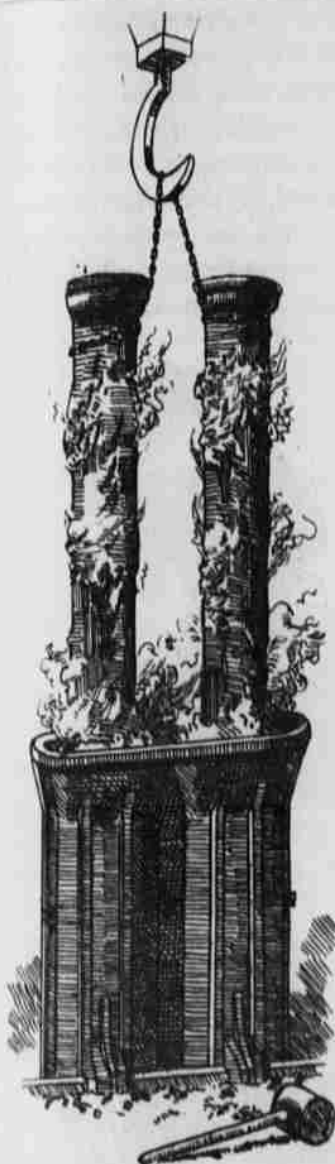
DRAWING NEWLY-CAST PIPES
