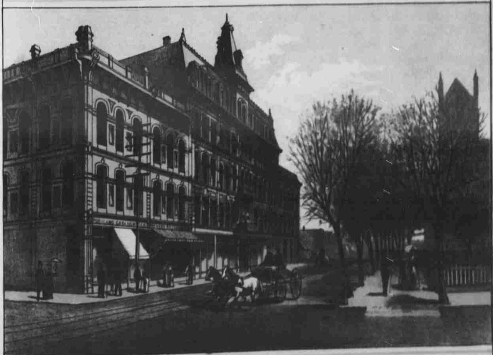
THIRD STREET, SOUTH FROM STARK,
