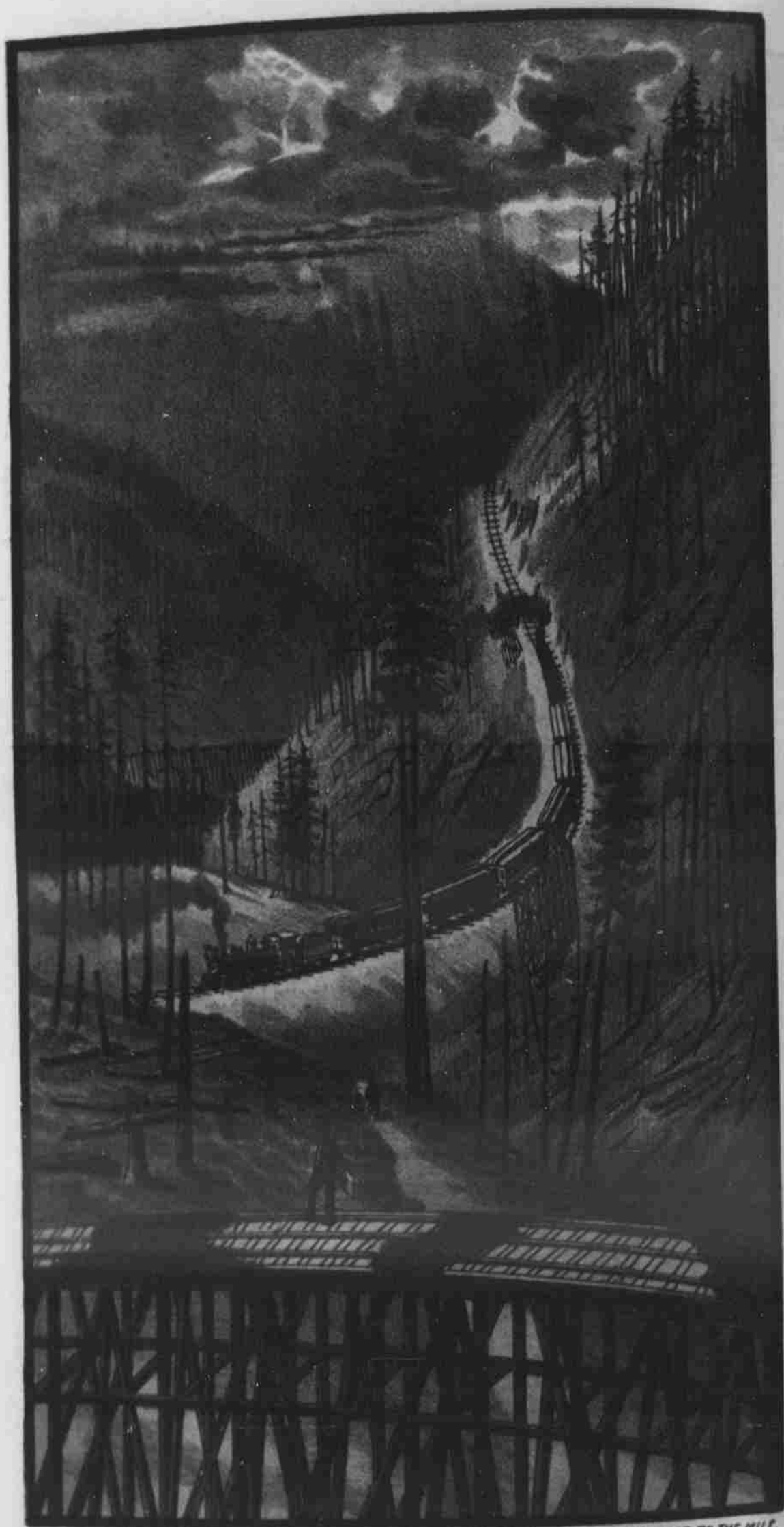
ACROSS "THE SWITCHBACK" FROM TACOMA. THE LONG PULL, 296 FEET TO THE MILE.
