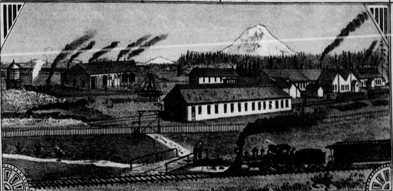
NORTHERN PACIFIC RAILROAD SHOPS.
