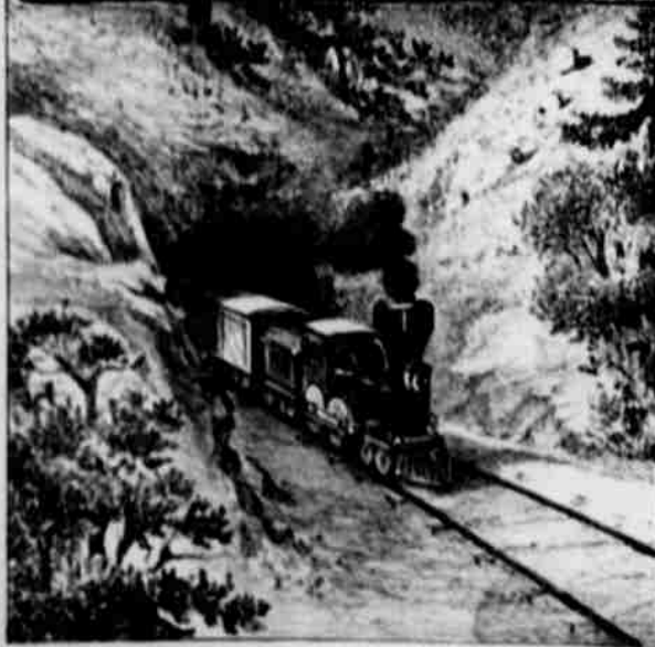
TUNNEL NO. 3 CANADIAN PAC. R. R.
