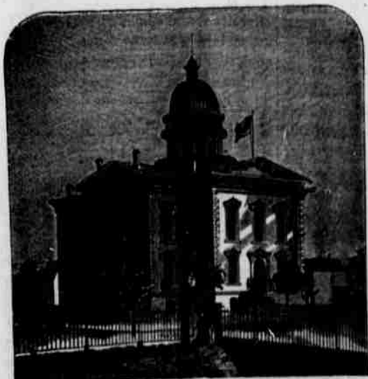
MULTNOMAH CO. COURT HOUSE—Portland, Oregon.
