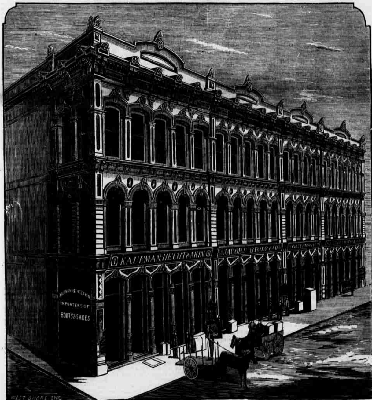
NORTH FRONT STREET, BETWEEN A AND B, PORTLAND.—Photo by A. H. Walzen.
