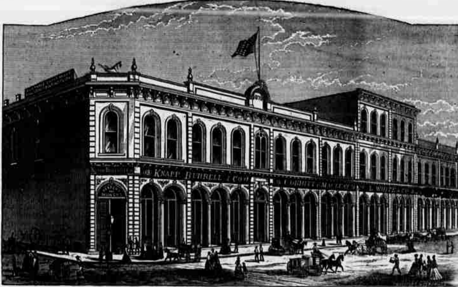
WEST SIDE FRONT STREET, BETWEEN VINE AND ASH, PORTLAND.
