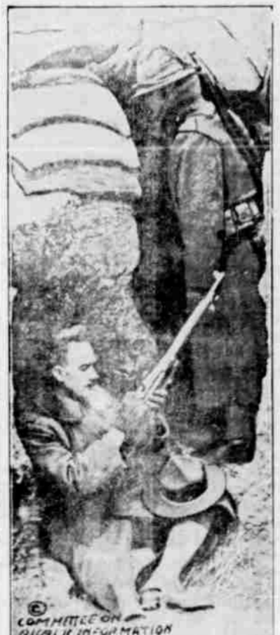
A view of an experimental trench showing an entrance to an underground passage. These warrens are constructed in all seriousness and the boys realize something of what a labor on the
