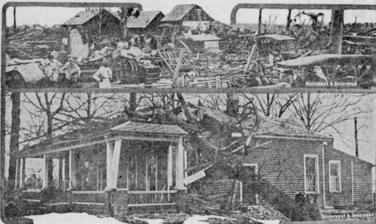
The cotton mill district of La Grange was almost entirely overturned by the recent tornado. The homeless were forced to make their beds among the wreckage. The lower picture shows an immense hole torn in a house by the tree.
