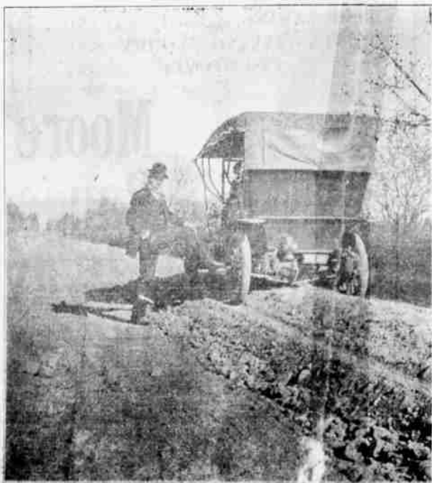
SNAPSHOT SHOWS COUNTY COURT'S METHOD OF ROAD-BUILDING. BROKEN ROCK DUMPED IN CENTER TO HEIGHT OF SEVERAL FEET.
