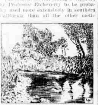
UNLINED CANAL. (Showing vegetation.)
