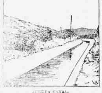
ALBERTA CANAL. (Showing with cement mortar.)
