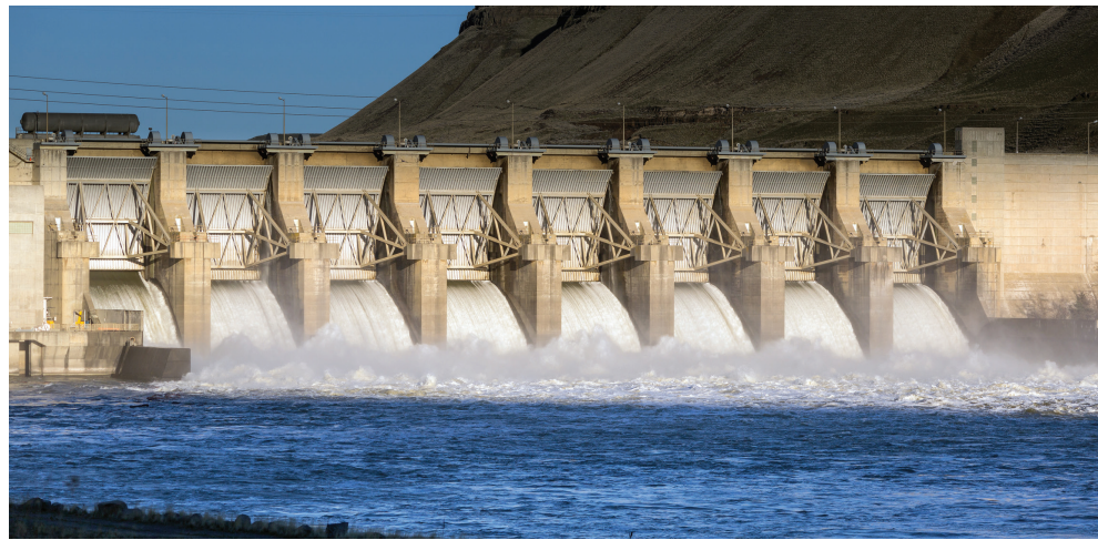
The spillway at Lower Monumental Dam in Washington on the Snake River.
