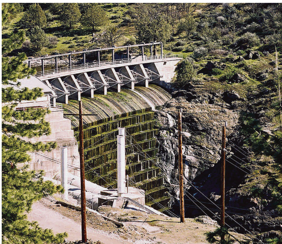
Copco No. 1 Dam on the Klamath River near Hornbrook, Calif., is one of four dams slated for removal.
