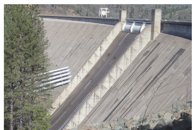
Capital Press File The U.S. Energy Information Administration projects a sharp decline this summer in the amount of electricity generated at Shasta Dam and other hydropower facilities in California.
