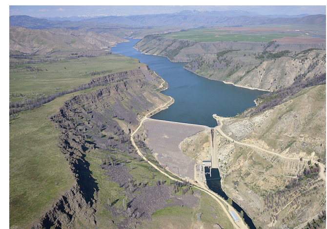
U.S. Bureau of Reclamation Anderson Ranch Dam in Elmore County, Idaho.
