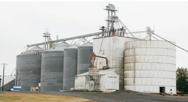
Matthew Weaver/Capital Press The CHS grain elevator in Rockford, Wash.
