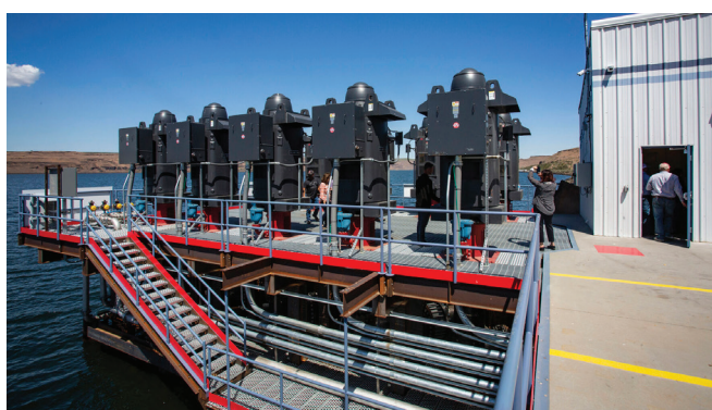
The East Project irrigation system pump station along the Columbia River near Umatilla, Ore. A similar facility is proposed to pump water from Lake Billy Chinook to help Jefferson County, Ore., farmers.
