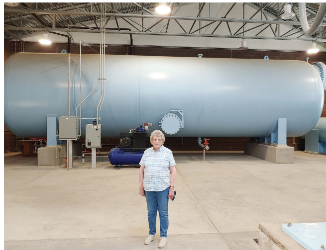
Alice Parker in front of the surge tank in the EL47.5 pumping station, the East Columbia Basin Irrigation District’s newest water delivery system.
