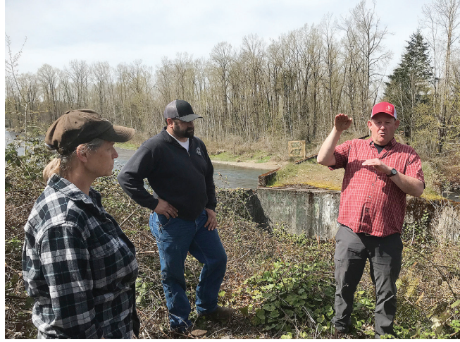
From left, neighbors Georgia Baker, Jason Paolo and Ken Baker stand on an old bridge over the Molalla River that's long been an attractive nuisance. Critics worry about a proposal to turn the crossing into part of a recreational trail.
