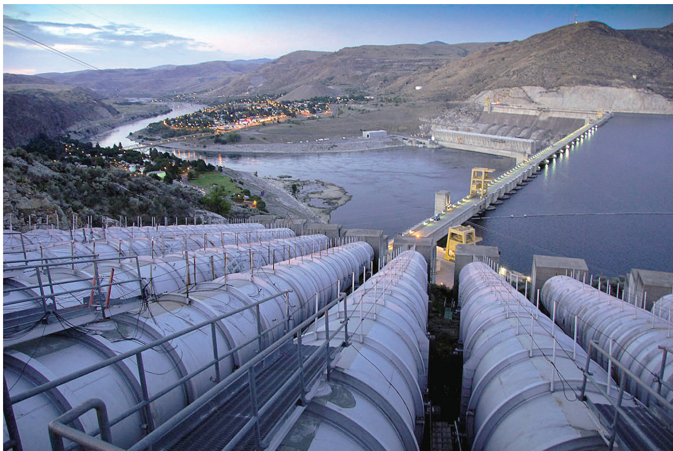
The John Keys Pump Generation Plant intakes at the Grand Coulee Dam. The 12 pumps send water from the Columbia River to Banks Lake and 670,000 acres of farmland in the Columbia Basin Project in Central Washington state. Work is underway to provide more water to farms and cities in the region.
