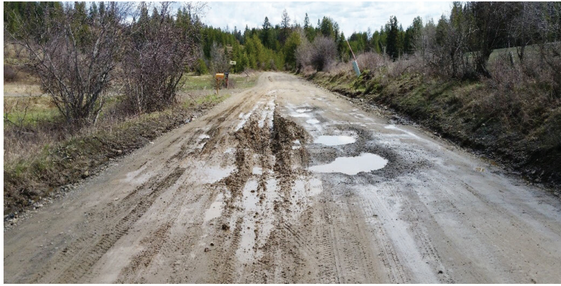
The road before any work was done.
