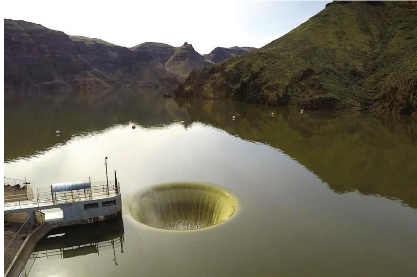
Bureau of Reclamation The "glory hole" at the Owyhee Reservoir funnels excess water into the spillway and into the river below the dam.
