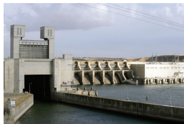
Associated Press File The Ice Harbor dam near Burbank, Wash.
