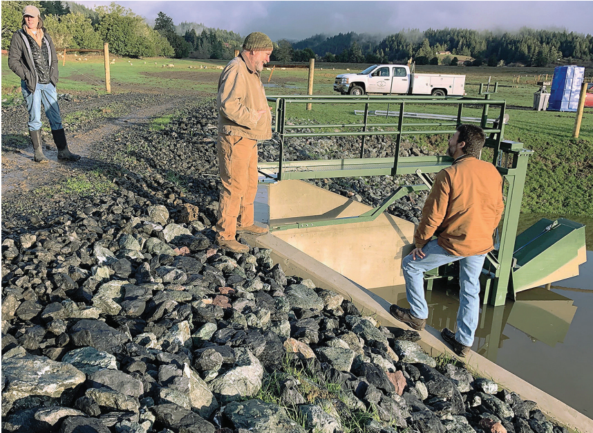
Gail Oberst/For the Capital Press Leo Kuntz, center, at the Seestrom Creek project on the Coquille River, has developed modern tidegates that can maintain both pastures and salmon habitat. Left is Melanie Dunne of the Coquille Watershed Association. Right is Chris Claire, ODFW biologist.
