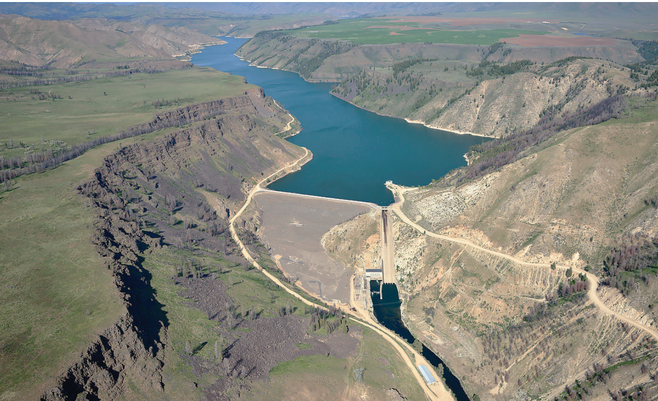
Bureau of Reclamation Anderson Ranch Dam is 456 feet tall and is on the South Fork of the Boise River, 28 miles northeast of Mountain Home, Idaho.
