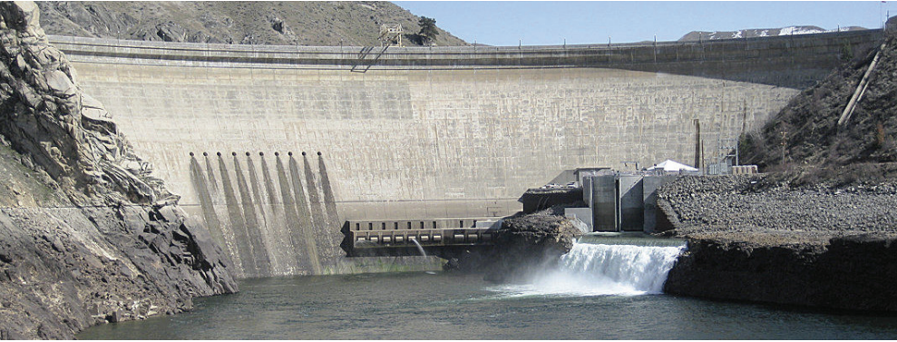
Boise Project Board of Control Repairs to three Arrowrock Dam gates took three days.
