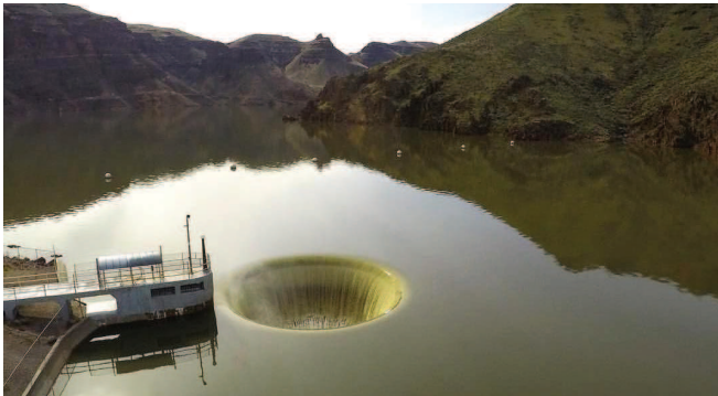
Courtesy Bureau of Reclamation The ‘glory hole’ at the Owyhee Reservoir funnels excess water into the spillway and out into the river below the dam.
