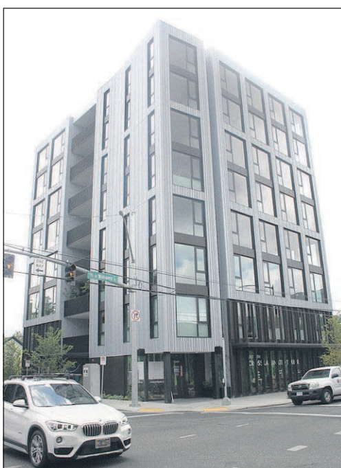
Carbon 12, an eight-story condominium building in Portland, Ore., is made with mass timber.
