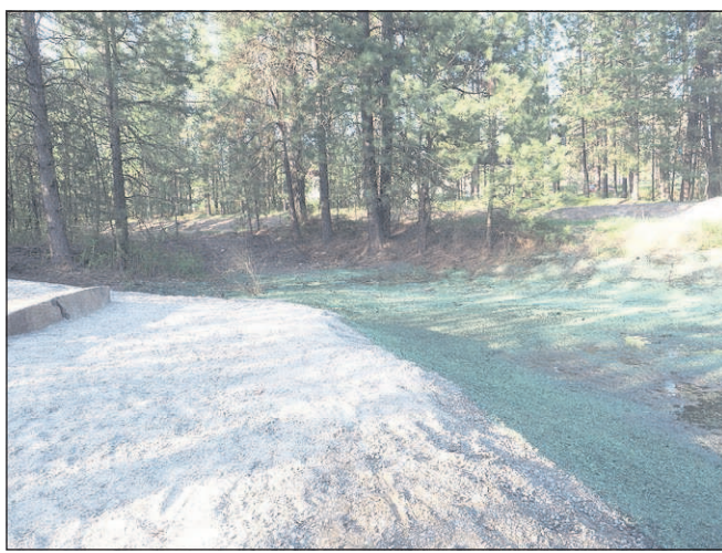
A new bio-infiltration swale at the University of Idaho Coeur d'Alene Center gathers and filters storm water before it enters the nearby Spokane River.
