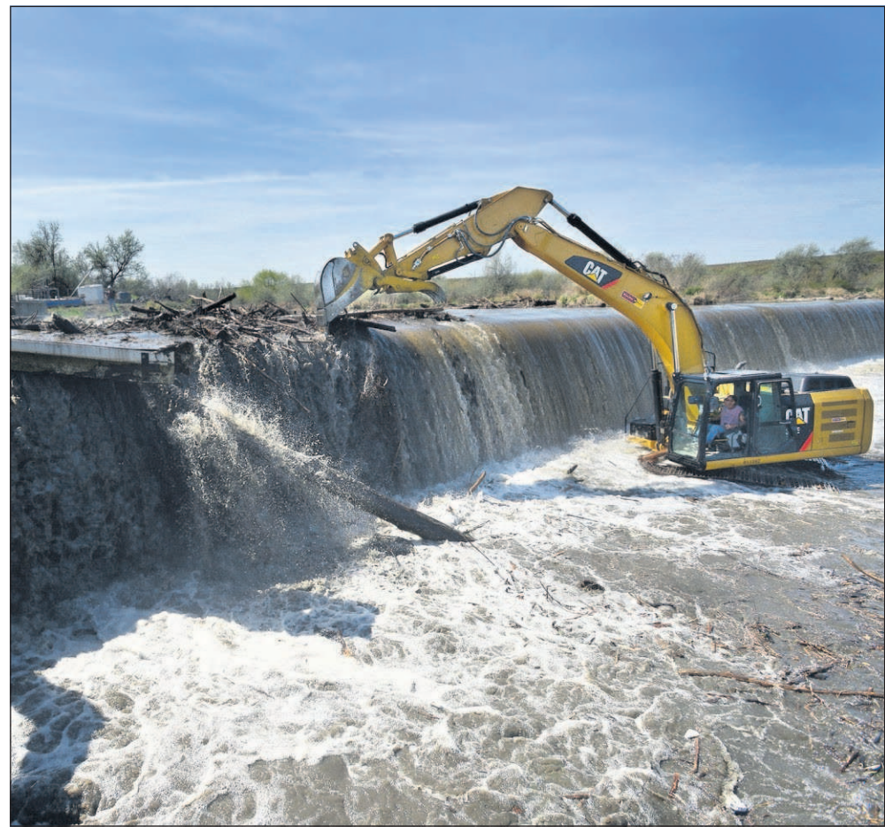
EO Media Group File An excavator breaks a log jam in April 2013 above the Three Mile Dam on the Umatilla River north of Hermiston, Ore. The Oregon Water Resources Department is considering seeking tougher dam inspection laws.
