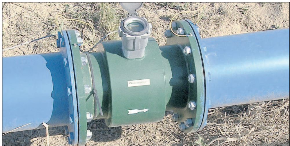
Idaho Department of Water Resources
