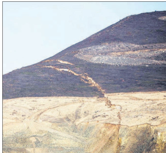
Associated Press A widening crack in Rattlesnake Ridge south of Union Gap, Wash., threatens to precipitate a massive landslide that could block Interstate 82 and the Yakima River. Authorities have urged about 50 people to evacuate.
