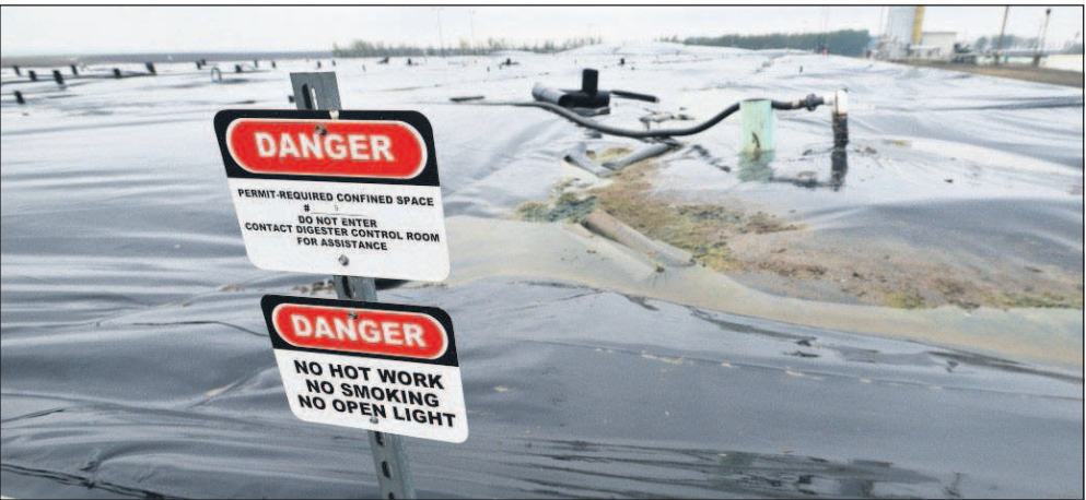
EO Media Group File A methane digester collects gas from decomposing cow manure at a dairy and uses it as fuel to generate electricity. Such generators could also produce carbon credits for Oregon farmers under “cap-and-invest” proposals considered by Gov. Kate Brown and the state legislature.
