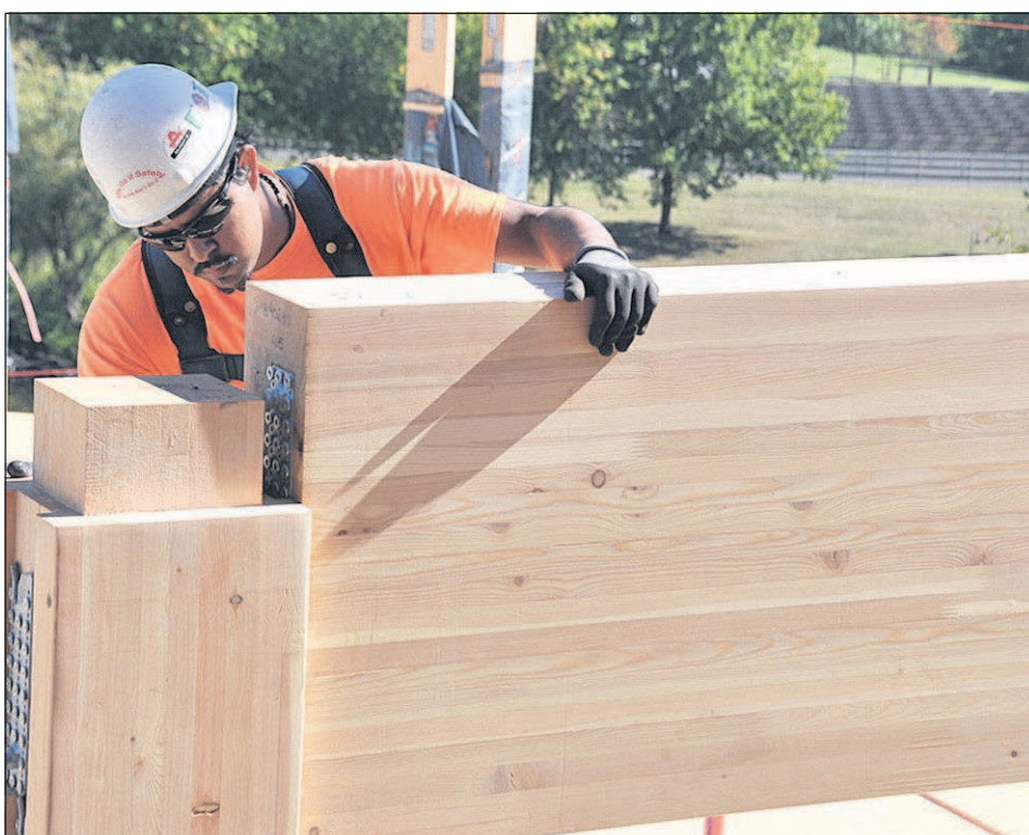
A worker guides a glulam beam into place Oct. 3 during construction of the First Tech Credit Union headquarters building in Hillsboro, Ore. The building, which will be five stories tall and include 156,000 square feet of office space, is believed to be largest U.S. structure so far built using advanced lumber products such as cross-laminated timbers (CLT) and glulam beams, posts and flooring. Advocates believe such wood products can replace concrete and steel in modest high-rises, and revive Oregon’s timber industry.
