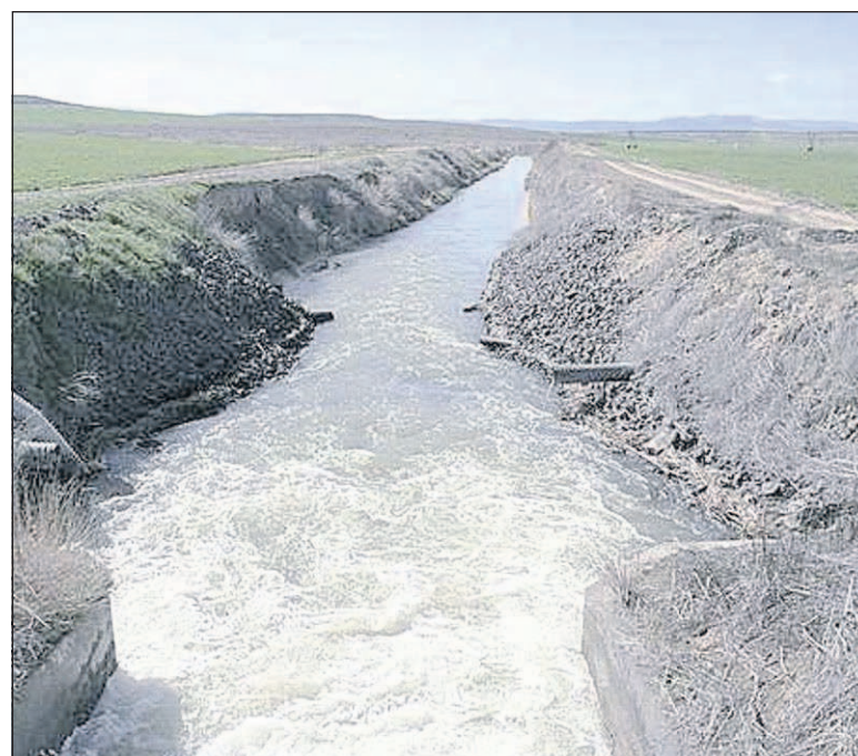
A canal brings federal surface water to Grant County in Central Washington. A Grant County farmer has been ordered to stop irrigating more than 500 acres with groundwater. Ecology says the groundwater right's place of use couldn't be changed because federal surface water is available.
