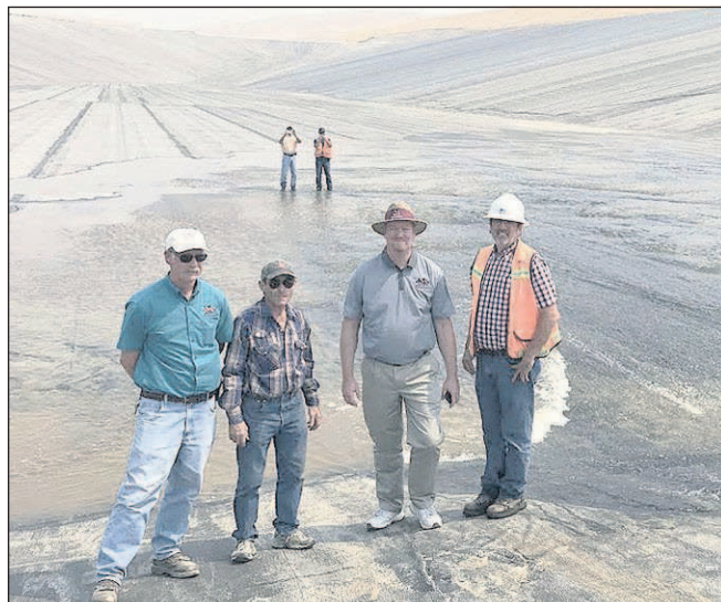
Courtesy Roza Irrigation District
