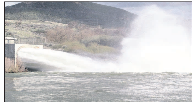
Sean Ellis/Capital Press Water is released April 14 from Lucky Peak Reservoir on the Boise River system for flood control.
