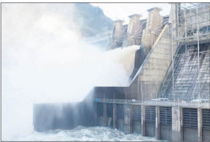
Courtesy of Idaho Power
