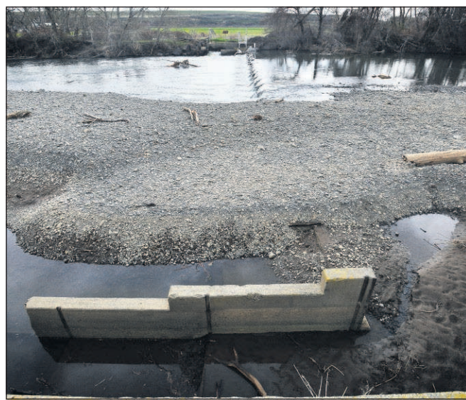
A large gravel bar washed over nearly half of the Dillon Diversion Dam on the Umatilla River outside Echo, Ore., in March 2014. The dam could be removed as early as next year.
