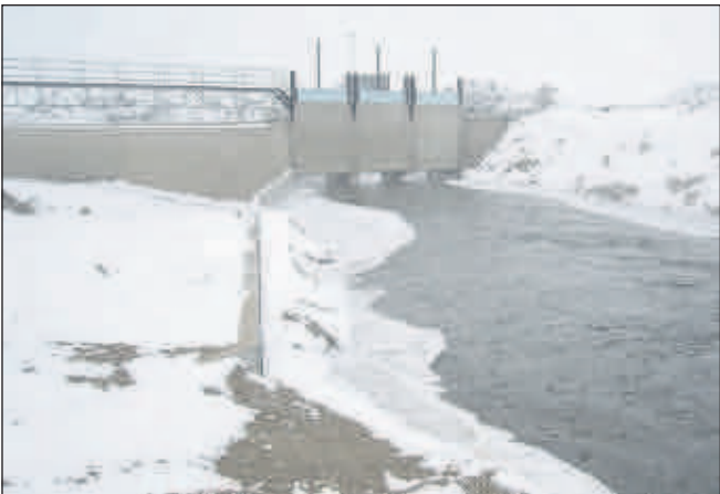
Courtesy of Idaho Department of Water Resources Water flows through the new Milepost 28 bypass around a hydro plant within the Milner-Gooding Canal, built to increase the state's aquifer recharge capacity. A concurrent resolution introduced in the Idaho Senate would enable legislators to provide their blessing to the 2015 settlement agreement between groundwater pumpers and surface water users in the Eastern Snake Plain Aquifer.
