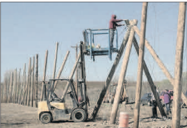
Dan Wheat/Capital Press A worker fastens trellis wire to poles about 15 feet above the ground for a new hop planting at a farm between Prosser and Benton City, Wash., last March. The planting was postponed because of drought. Fields like this will be planted this year.
