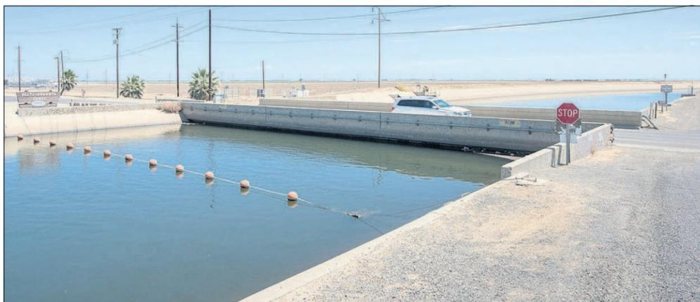
A bridge over the Delta-Mendota Canal in Firebaugh, Calif., in the western San Joaquin Valley nearly touches the water because of subsidence of land caused by groundwater pumping. A California Water Foundation study asserts flooding farmland to recharge aquifers could curb subsidence by as much as 20 percent.
