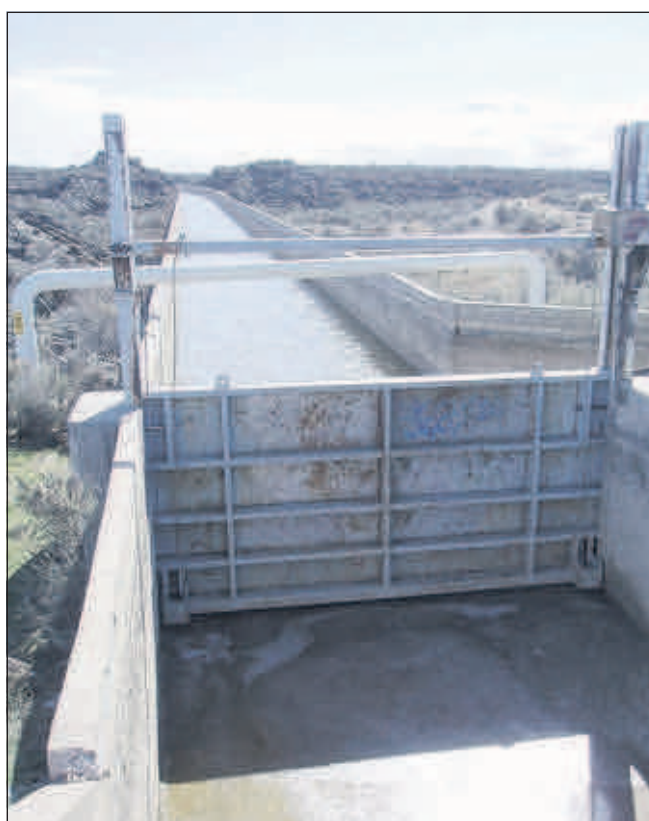
Courtesy of Idaho Department of Water Resources
