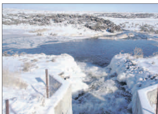
Courtesy of Idaho Department of Water Resources
