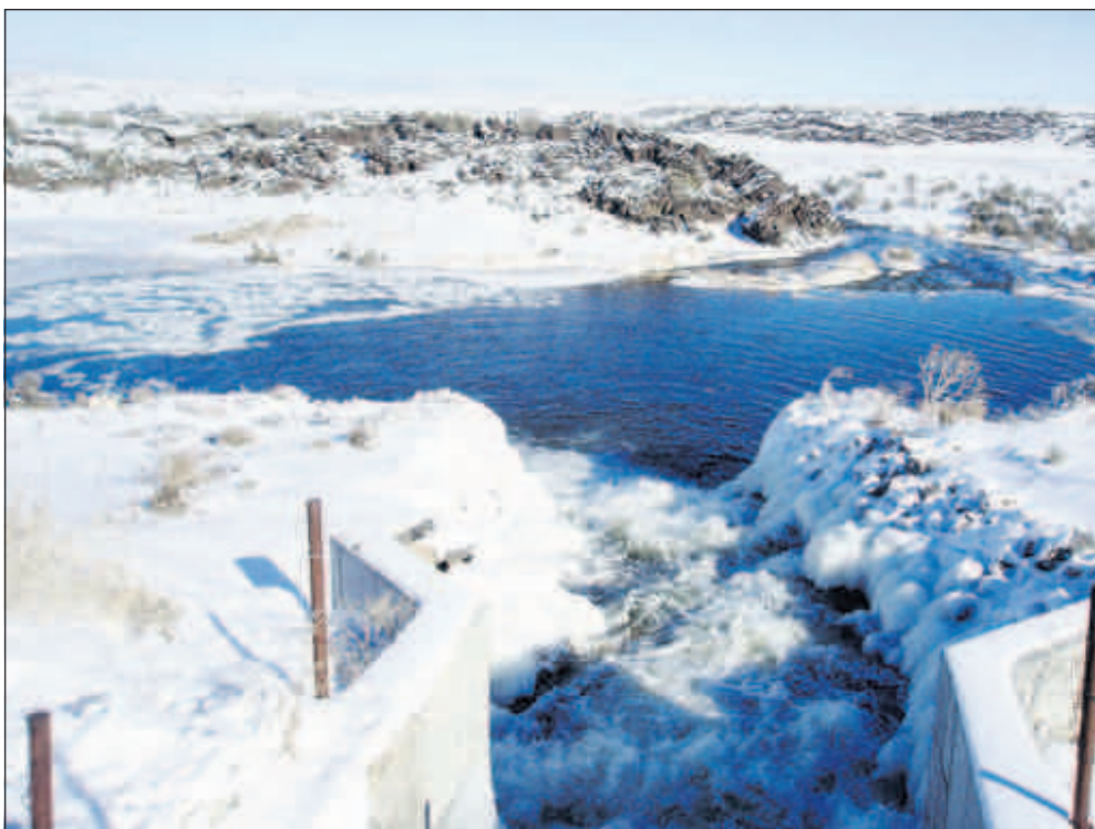
Submitted by the Idaho Department of Water Resources Winter aquifer recharge is conducted recently at American Falls Reservoir District No. 2’s Milepost 31 recharge site. A work group has been assigned to draft a bill for the Idaho Legislature to implement an aquifer recharge credit system for the Eastern Snake Plain.
