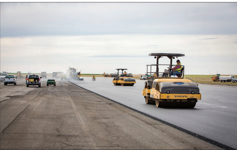
East Oregonian, File Rollers compact the asphalt of the primary runway in April 2020 at the Eastern Oregon Regional Airport in Pendleton. Oregon U.S. Sens. Ron Wyden and Jeff Merkley announced Monday, July 25, 2022, that the Pendleton airport is receiving almost $5 million in federal grant funds to reconfigure a runway.
